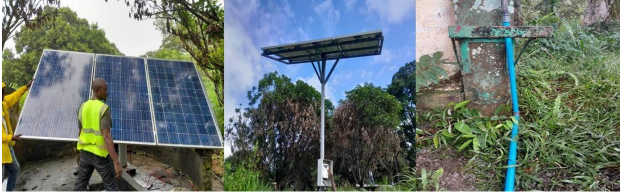
Figure F2. Photos of the installation of the solar submersible machine at MLWERC
