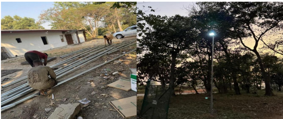
Figure F3. Photos of the installation of 12 solar street lights at MLWERC
